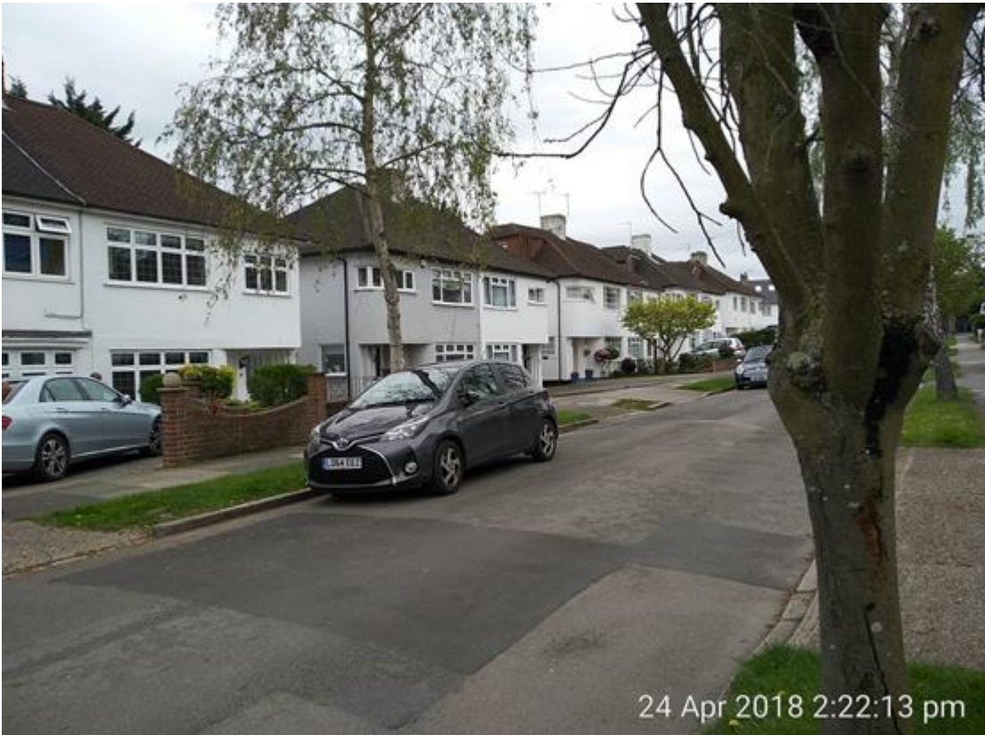
Street context- opposite side towards south-west
